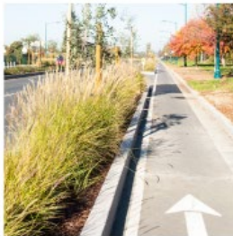
Protected bike lane
